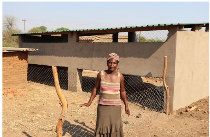
Sibongile is pictured with her new goat housing structure, made possible by the match funding initiative. The small brick pen on the left is what was previously used to house her goats. PHOTO: ActionAid
